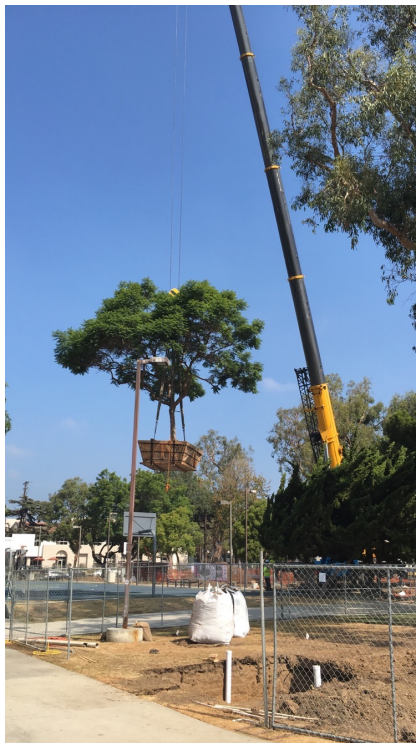
Onsite Jacaranda relocation as part of Reed Park landscape improvement & exercise area retrofit.
